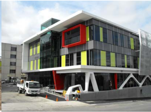
▲ Launceston General Hospital, new energy efficient building
