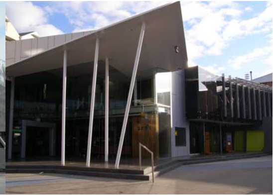
▲ 2 Salamanca Square, 4 Green Star rated redevelopment
