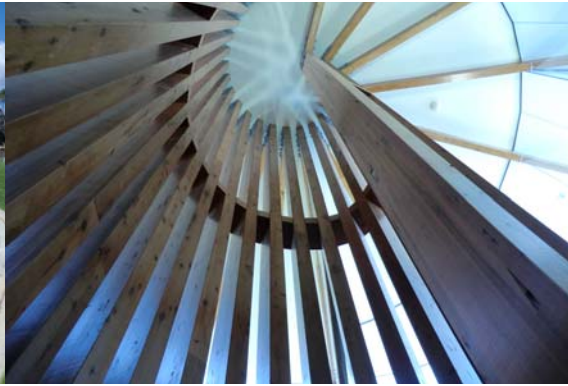
▲ Administration Block main structural timber support
